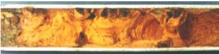
Pitting and hollows (Photo: CEBTP)
