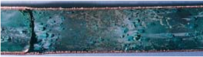
Internal corrosion (Photo: CEBTP)
